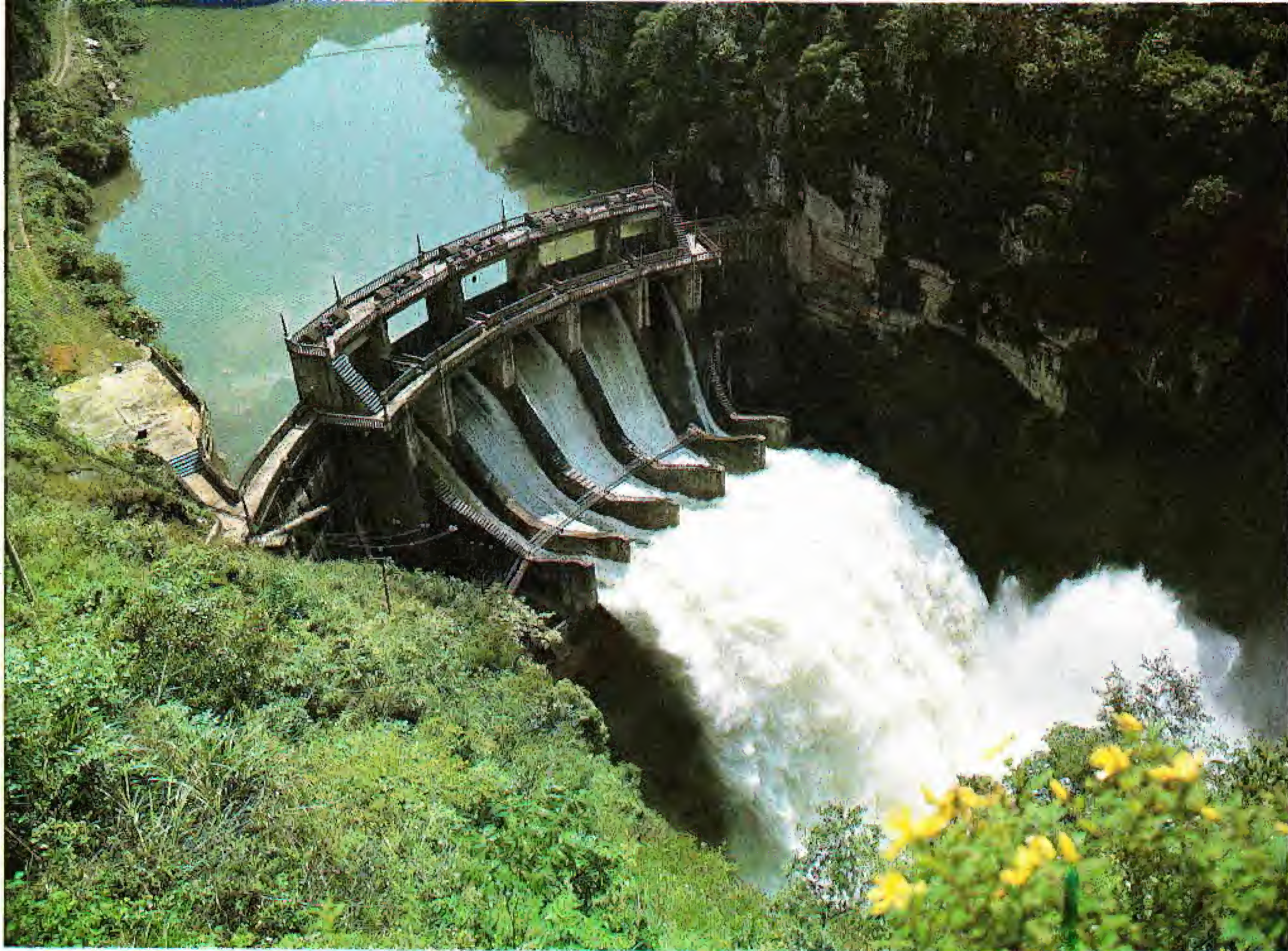
The Xiuwen power station—the third one down on the Maotiao River. Li Zhusheng and Peng Kuang
